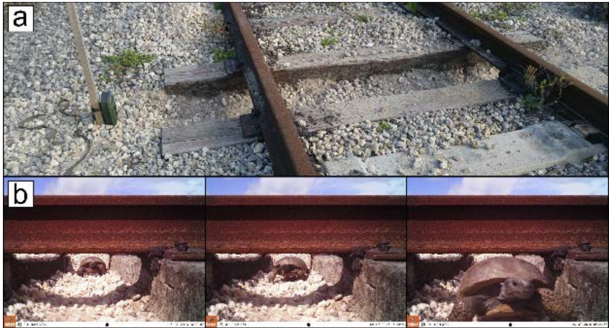
Figure 9: (a) The trench dug underneath the rails and between the railway ties. A game camera faces the entrance/exit on the west side of the railway to photograph Gopher Tortoises passing from one side to the other. (b) A series of pictures of a single Gopher Tortoise moving from the east side of the tracks to the west side.
